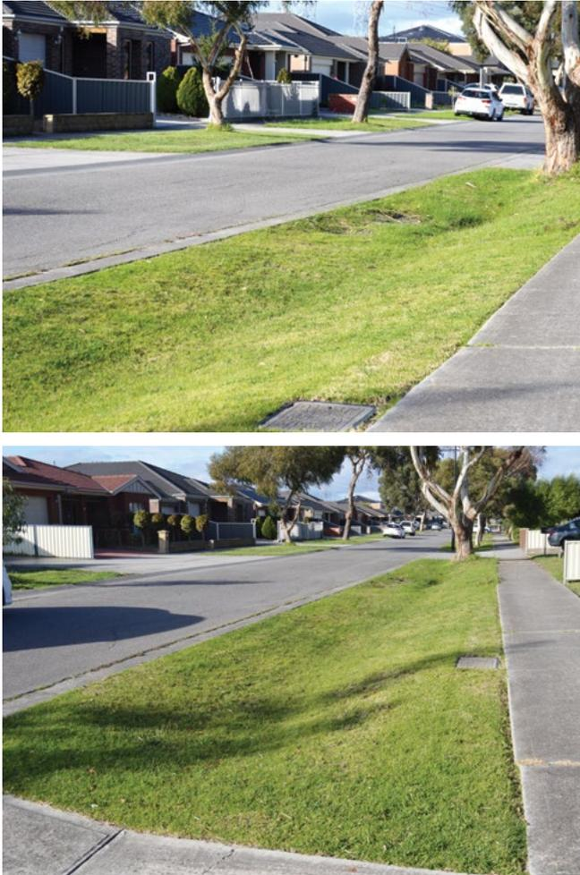
**Figure 4** Examples of drainage swale/channels.
